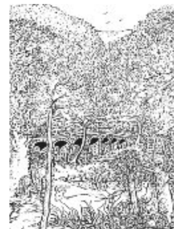
Seven Arches Aqueduct 1840
