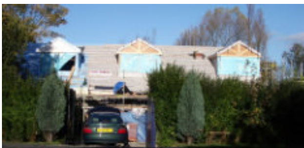
d. Work in progress on Farrar Lane
