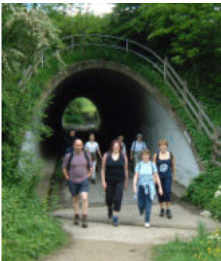
A6120 Ring Road, Adel Underpass
