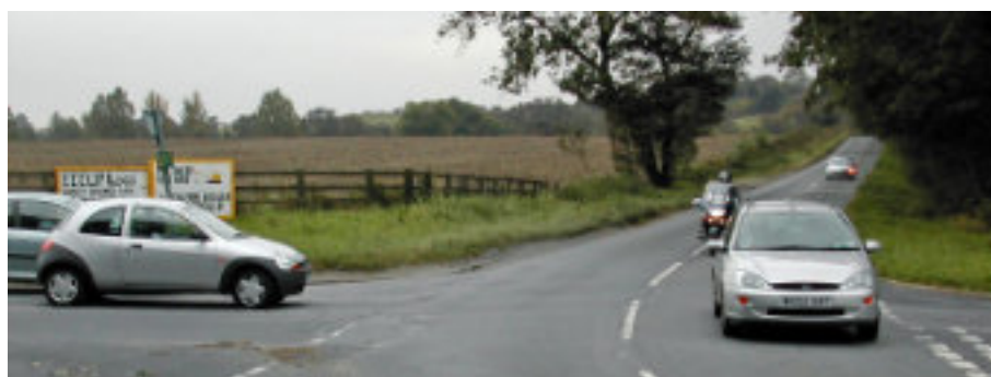
Five Lane Ends
