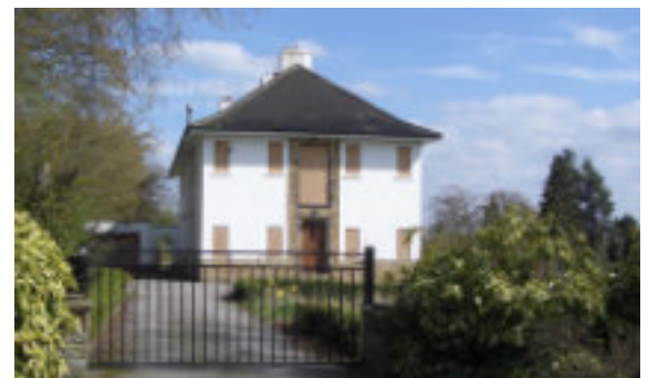
Boarded up Townend before demolition
