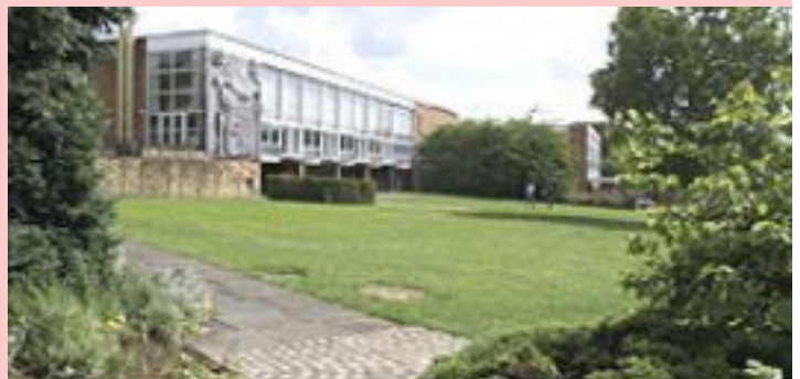
Bodington Halls of Residence
